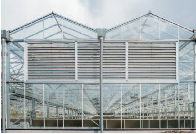
Supply of fresh air to the greenhouse
