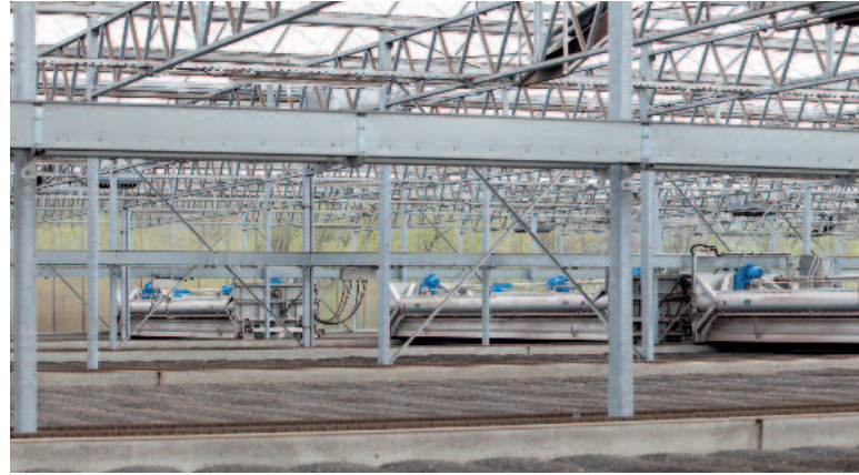
Parallel operation of HUBER Sludge Turner SOLSTICE® units
