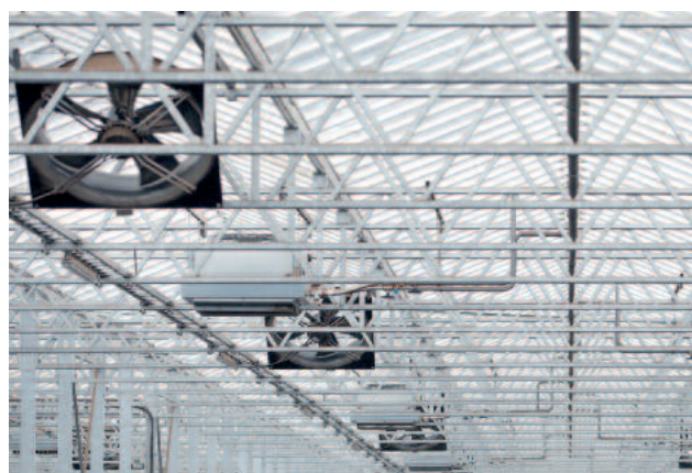
Recirculation air ventilators and optional air heaters
