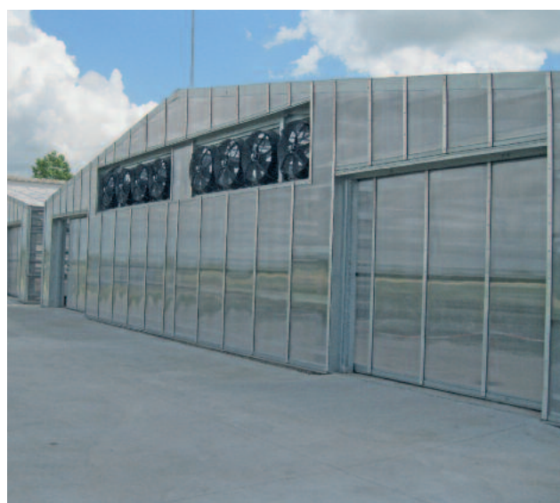
Exhaust air ventilators
