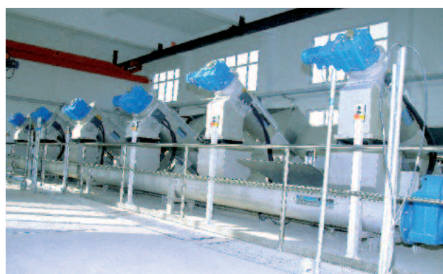
ROTAMAT® Membrane Screen RoMem units installed to protect a large downstream MBR plant
