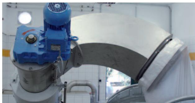
*Individually adapted installation with lateral screenings discharge directly into a container*
