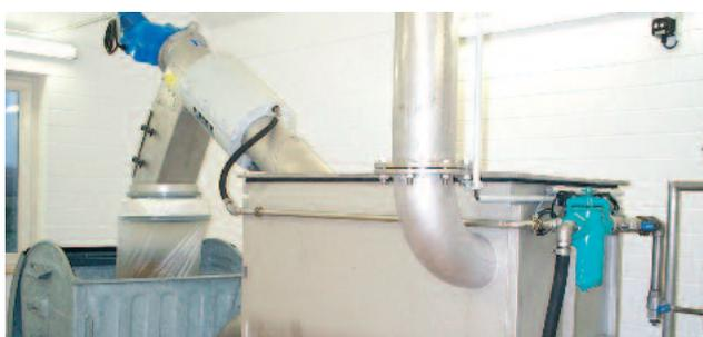
*Tank-mounted HUBER Rotary Drum Fine Screen ROTAMAT®...*
