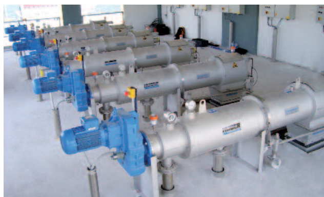
Sludge screening on WWTP Athens, Greece
