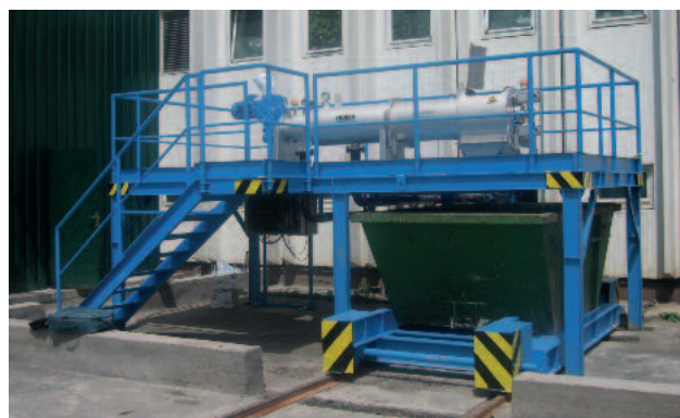
Outdoor installation of a HUBER Sludgecleaner STRAINPRESS®
