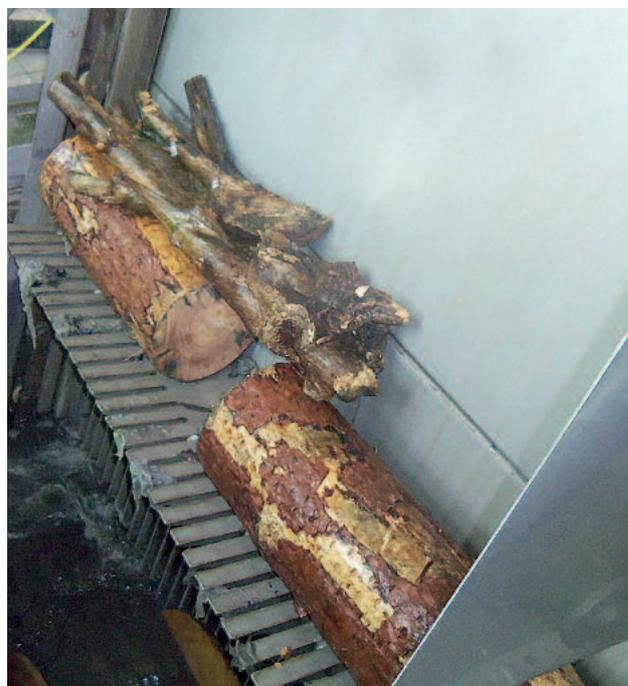
*The screen rack is cleaned by very robust high-capacity rakes. The number of cleaning rakes can be variably adapted, removal capacity is then adjustable. Even extremely bulky objects are reliably removed by the screen rakes and transported upwards out of the channel to the screenings discharge.*
